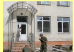
The Window Replacement Project Finished!! Svalyava, Ukraine
